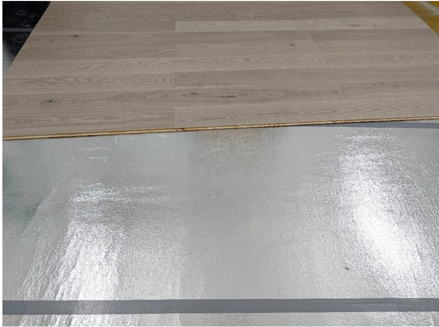
Figure 3: mounting situation of insulating underlay and parquet flooring
